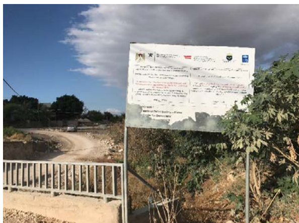
Figure 3 A section of agricultural road that was rehabilitated in Tubas cluster
